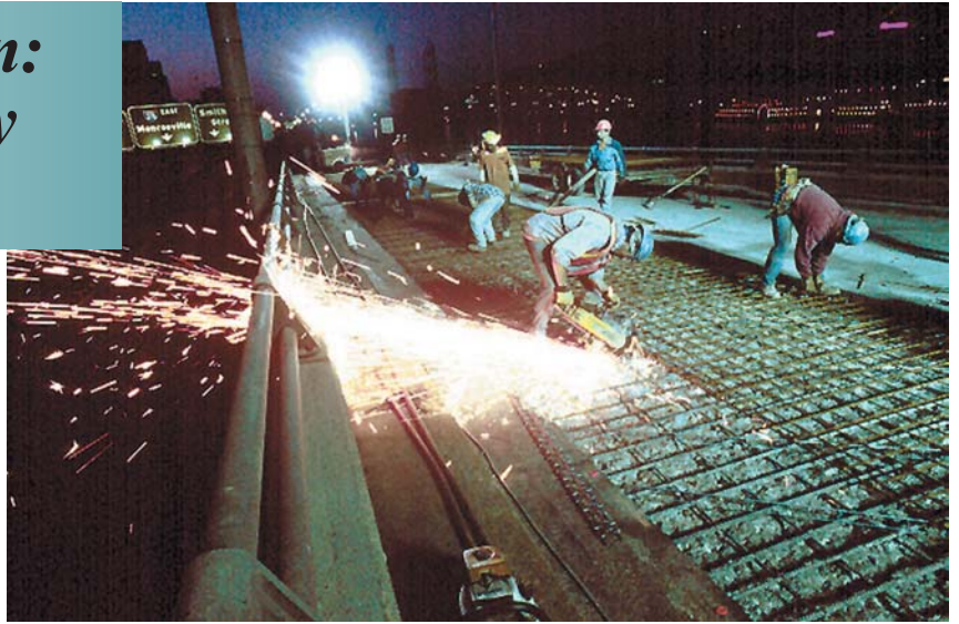
The challenge of refurbishing the Fort Pitt Bridge and Tunnel
