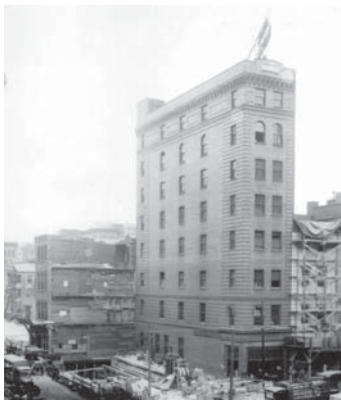
The Joseph Woodwell Company Building
