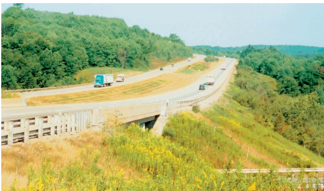
I-80 west-bound over SR 0338 looking West
