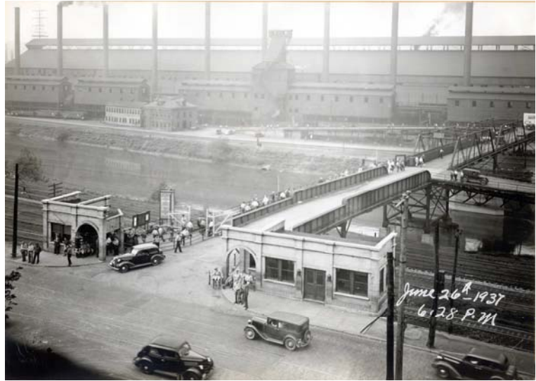
Former Steel Mill access bridge.
