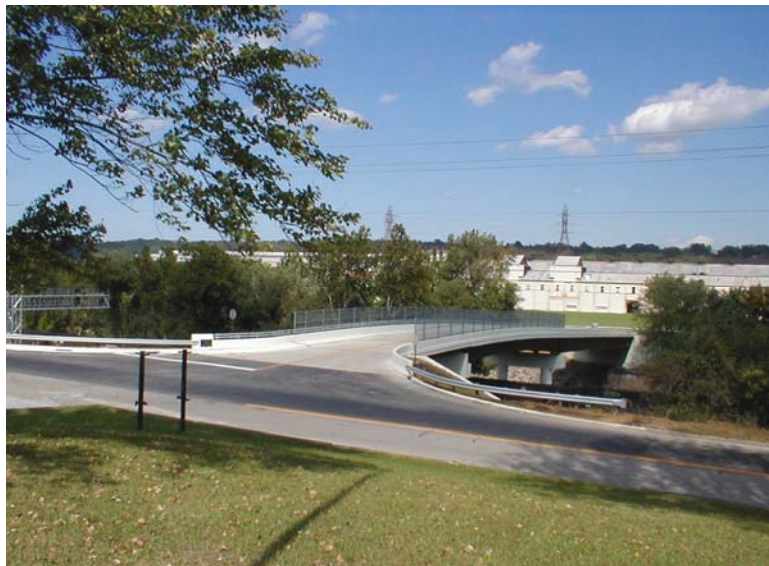
New "Steelworkers Bridge" at same site.
