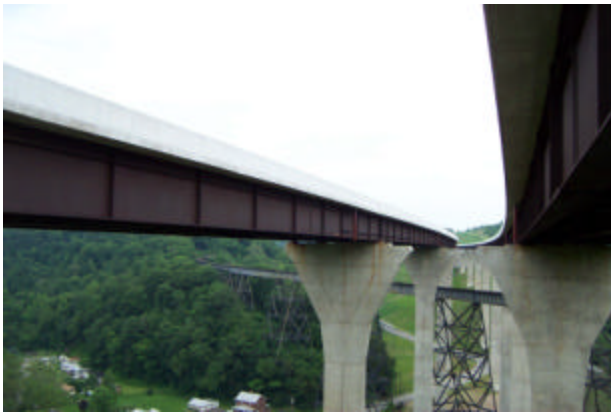
Figure 2 - Joe Montana Bridge on the Mon-Fayette Expressway
