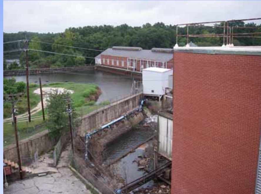
Rooftop view of Langdale Mill in Valley, AL
